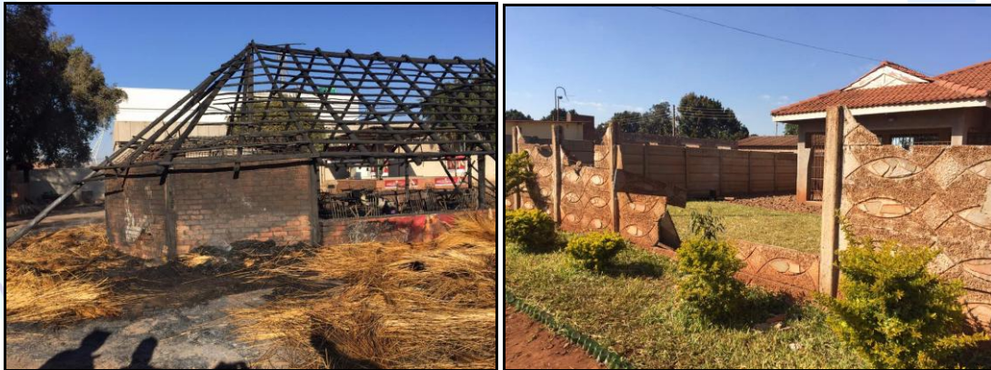
(Left) Duriro bar owned by Mudzuri was set ablaze while the home of Janjazi (right) was destroyed by suspected Zanu PF youths [picture by ZPP]
